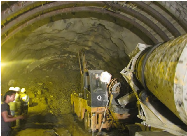
Head Race Tunnel
