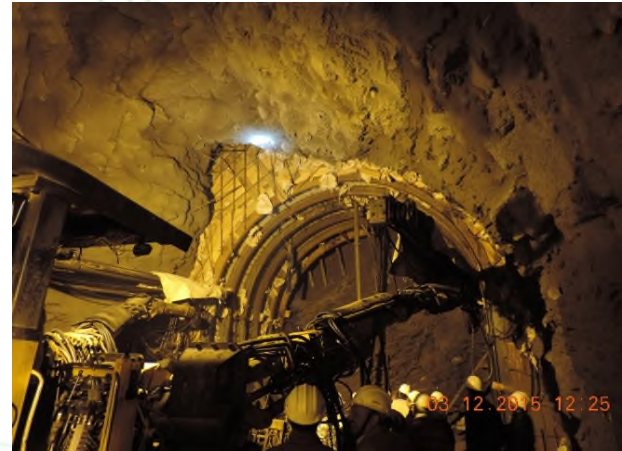
Head Race Tunnel
