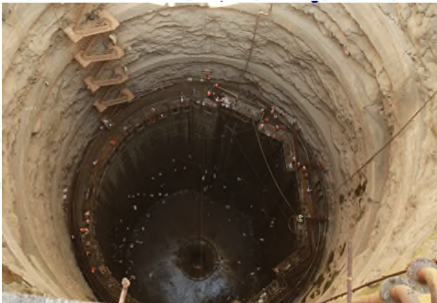
24.5 m dia. Surge Shaft
